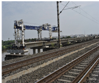
Construction at one of the sites of dedicated
