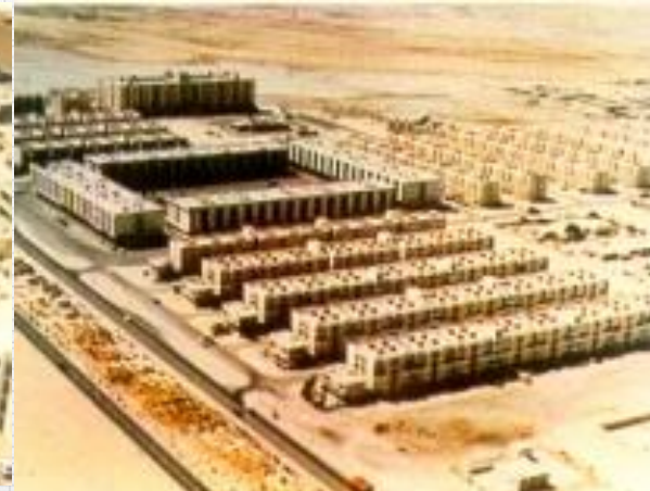
DUBAI : BUILDING COMPLEX, WITH ALL SERVICES IN THE GUSAIS AREA
