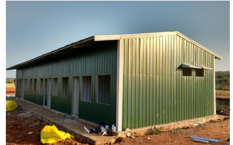
LABOUR SHED - HUBLI
