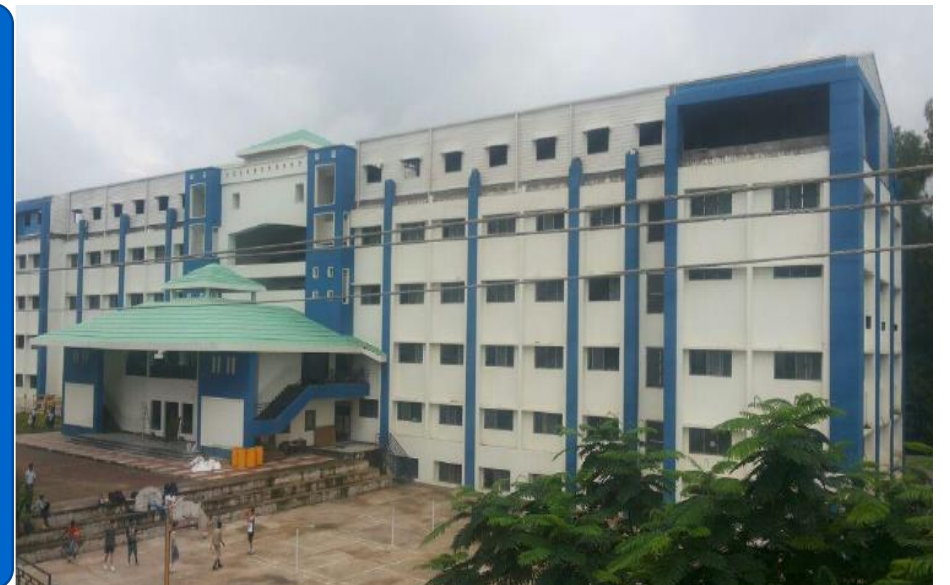
Roof top Class Rooms
