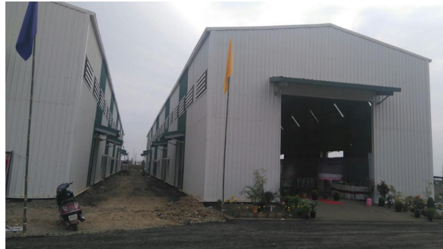
NIT IMPAL – WORK SHOP
