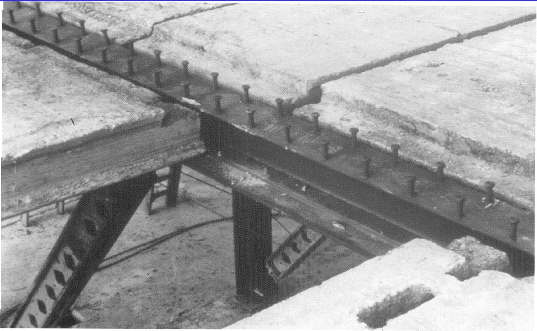
Slimflor beam with pre-cast slab
