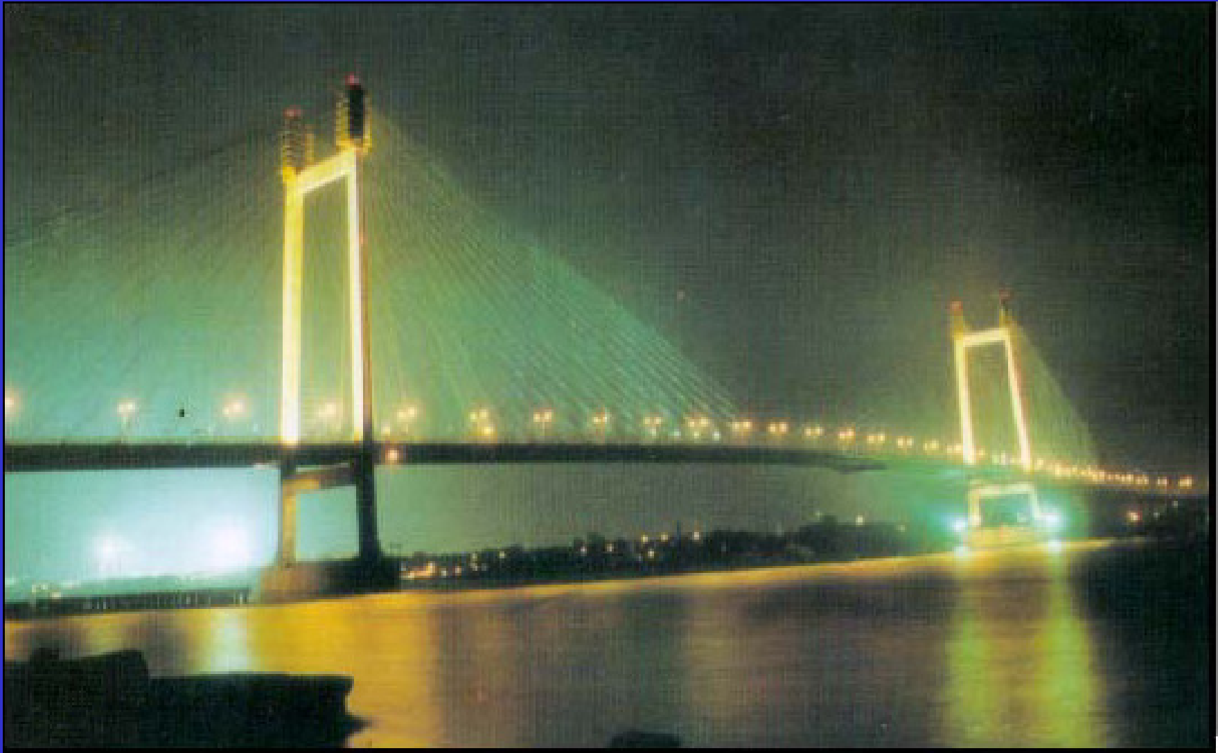
Fig.2 The second Hooghly cable stayed bridge
